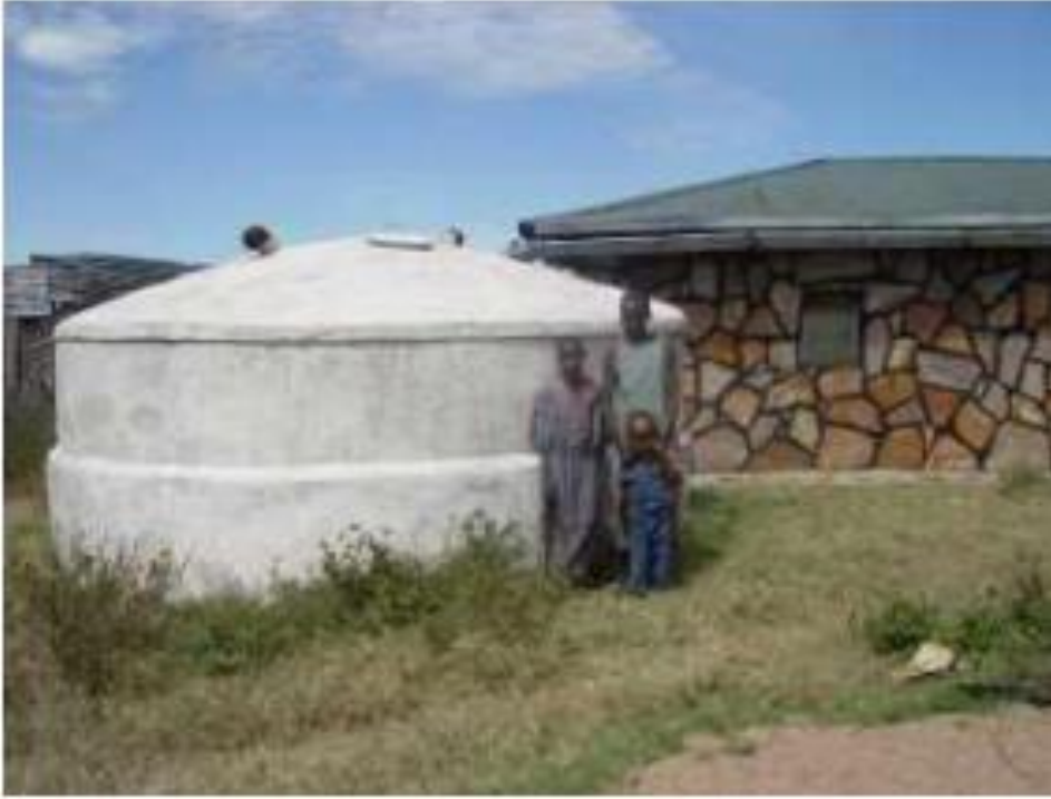
Figure III: Concrete Rain Water Storage Tank
